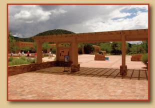
preventing some pollutants from reaching the aquifer. The joint material should adequately allow the passage of water to quickly drain, possess the structural capability to withstand traffic loads, and provide horizontal stability to the paving surface.
