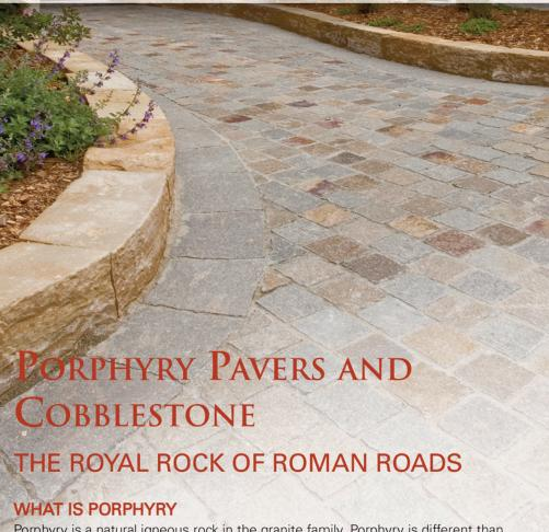
Porphyry is a natural igneous rock in the granite family. Porphyry is different than other granites, in that as it cooled from a sub-surface magma formation, seismic activity created fissuring allowing for rapid cooling, creating dense slabs of variable thickness with an even yet rough surface that does not become smooth, due to wear, or slippery when it rains.
