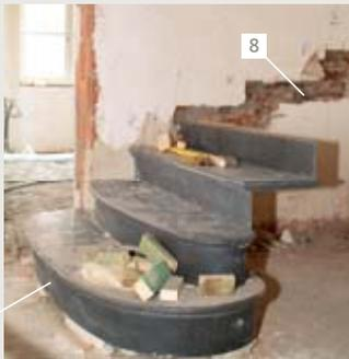
setting facing plaster. As the staircase gradually rises, bricks laid in the plaster come and wedge the step/riser assembly. A distribution vault made of brick comes and solidly fastens the staircase ending in a bottom vault, itself smoothed with plaster. The assembling of the bricks is designed in such a way that the overall assembly is self-supporting. The assembling of the steps and risers therefore determines the vault and not the opposite.
