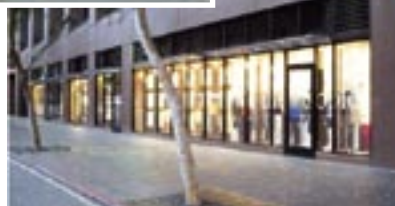
A false facade provides the appearance of a transparent ground floor at the Edward J. Schwartz Federal Building, San Diego, CA.
