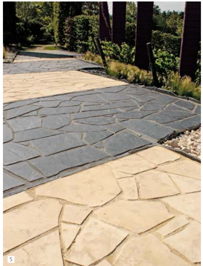
5 COLOURED JOINTS: The joints add the finishing touch to a paved area! Thin or thicker joints, the decision depends on whether you wish to create a traditional, contemporary or natural atmosphere. The colour is also a crucial point and it is worth giving it a lot of consideration before laying the stones. In this theme park where originality was a welcome feature, random bond or opus incertum provides an alternating pattern of shale and white stone. The joints harmonise with the stone for a strikingly graphic result.
